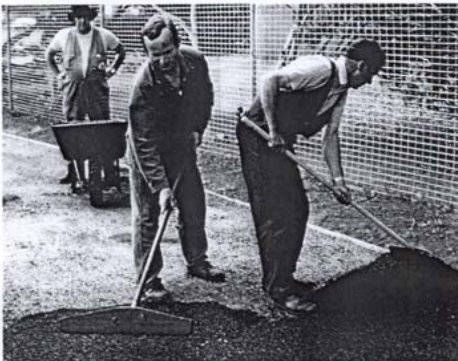
Workers lay tarmac on the Moonee Ponds bike path, Victoria, in 1985
