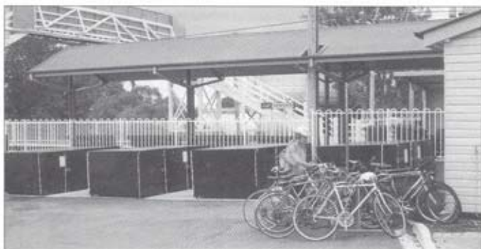
Free bicycle lockers at Sandgate Station, Brisbane. 540 bicycles are stored in lockers 20% to 30% of these cyclists previously parked their cars at the station.
