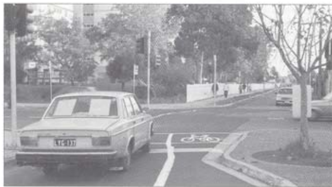
Turning a "RatRun" into a bicycle route. One way for cars, two way for bicycles. Alternate one way direction for cars to create discontinuity. Richmond, Melbourne.
