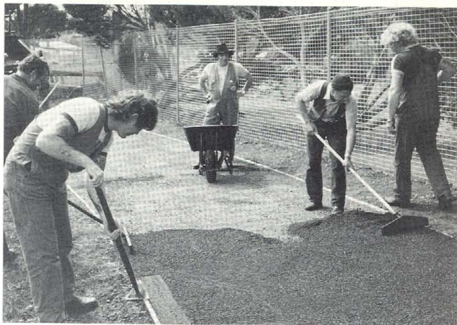
CEP workers laying tarmac on Moonee Ponds Creek bikepath, Victoria, 1984.
